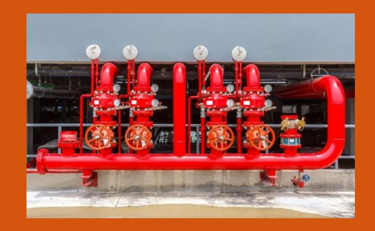
Fire Hydrant system is a mechanism where water is pumped, tapped off and released in the form of a jet through a nozzle to extinguish the fire.
